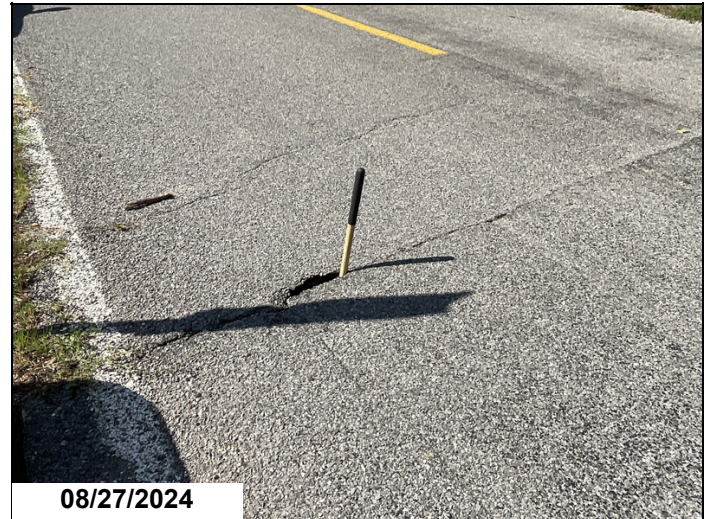
Roadway embankment at Bent 1, right lane, right wheel path, void in the embankment at the backside of the abutment below the asphalt. The void is 4' deep x 1' long x 2' wide.
