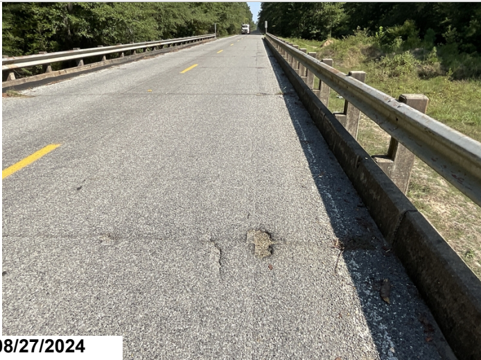
Right side several spans have spalls in the top flange.
