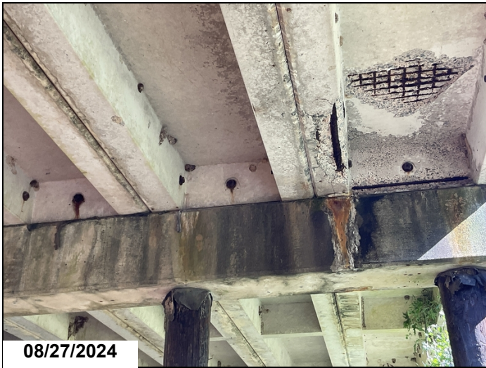
Span 3 Unit 7 back of Bent 4, 3LF exposed rebar CS3.
