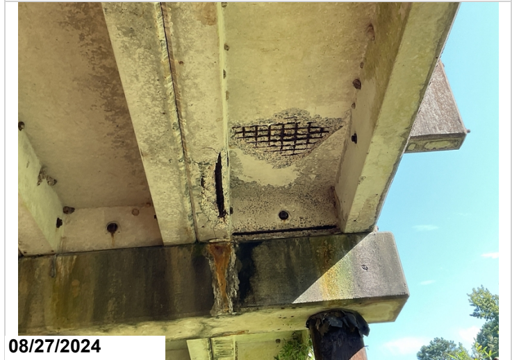
Span 3 Unit 7, under surface back of Bent 4, 2SF exposed rebar CS3.
