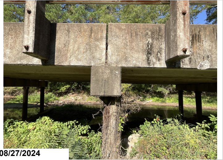
Bent 5, right end, Pile 5 is ahead of center of the cap, the units are centered on the cap. Bent 6, 7, and 8 are similar.
