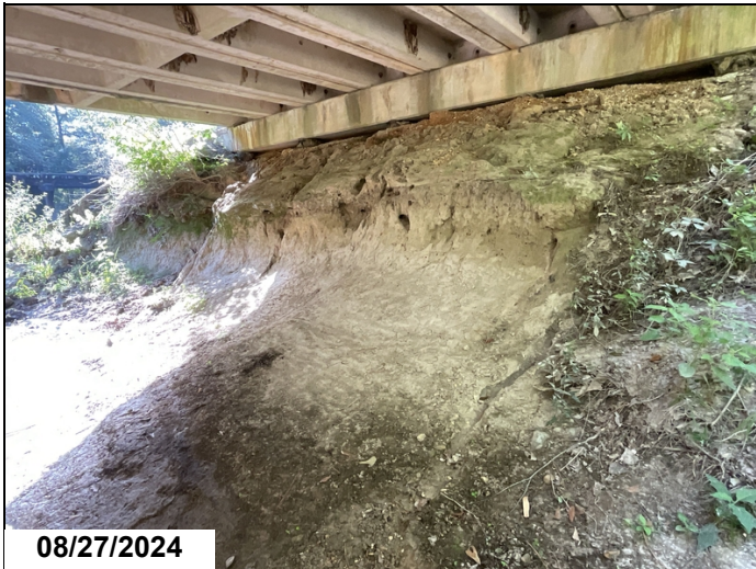
Bent 1, Embankment has settled 10" below the abutment allow erosion to cause the void behind the abutment.
