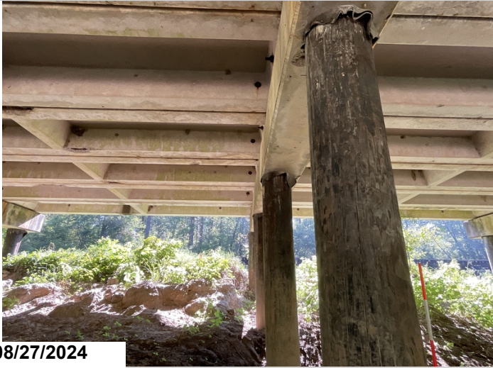
Bent 5, ahead side, Piles 2 - 5 get progressively farther ahead of center of the cap the further you look right.
